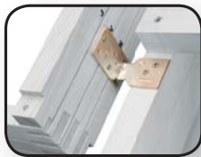
Installation on rafters
