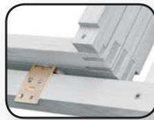
Installation on battens
