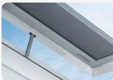
The servo-motor in electrically opened windows is positioned in the sash and is protected against adverse weather conditions such as rain and snow.
