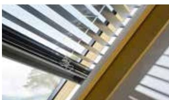
Side aluminium guide rails enable a complete shading of the room and keep the slats in line.
